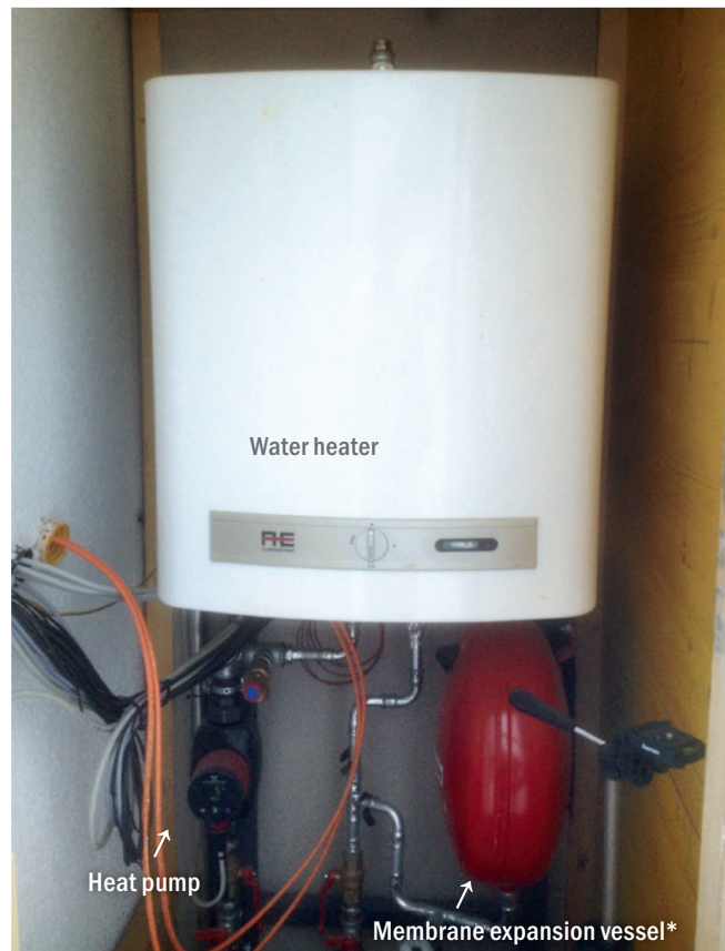
Equipment room with electric water heating
