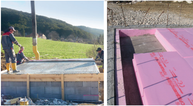
Concrete floor slabs with XPS insulation
