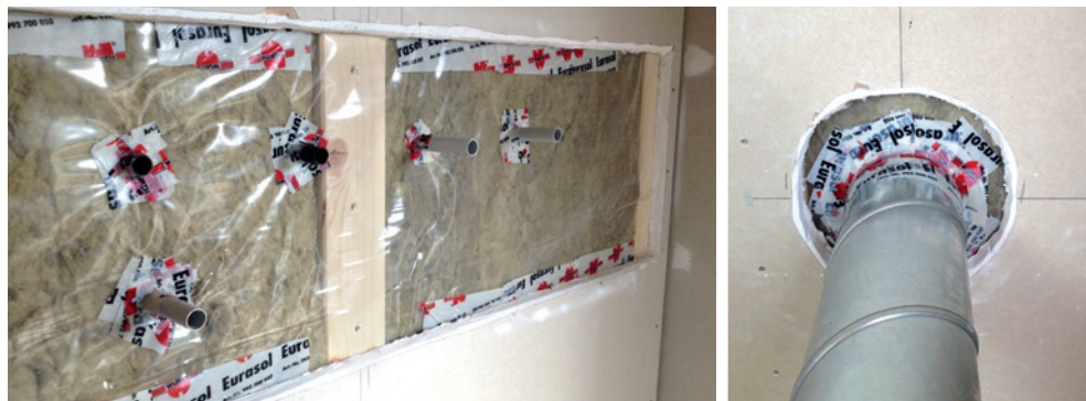
Installation of empty piping for the measuring sensors in the houses with wood frame construction
