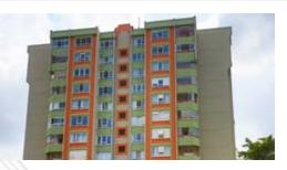
**Description:** Kardelen Sitesi is a renovation project of 3,500 m<sup>2</sup> in Ataşehir. In thermal renovation mineral wool insulation boards and new paint Baumit StarColor have been used.
