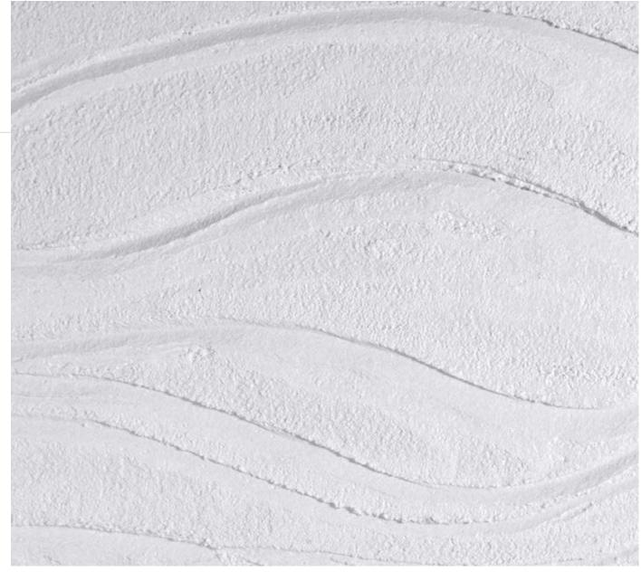
SNOW IMPULSE Brings dynamism to the wall Products: Baumit CreativTop Fine applied with trowel forming soft waves.
