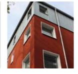
**Description:** The development dates back to the 1930s and features a brick faćade. The houses have been renovated acc. to the latest energy standards. An extensive colour concept was created for the energy-saving renovation of the faćade surface needing to fit to the intense colour of the existing clinker surfaces.
