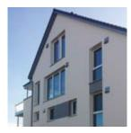
**Description:** Modern apartment building in wood construction with mineral wool insulation. Energy efficiency KFW 55. Fascina SEP02 roof plaster, painting with NanoporColor.
